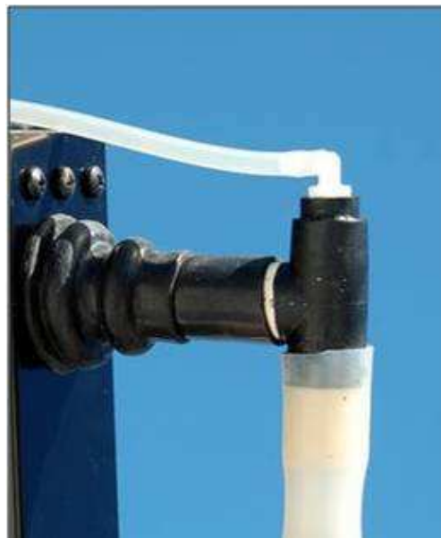
Figure 12: outlet plumbing with permanent vent
